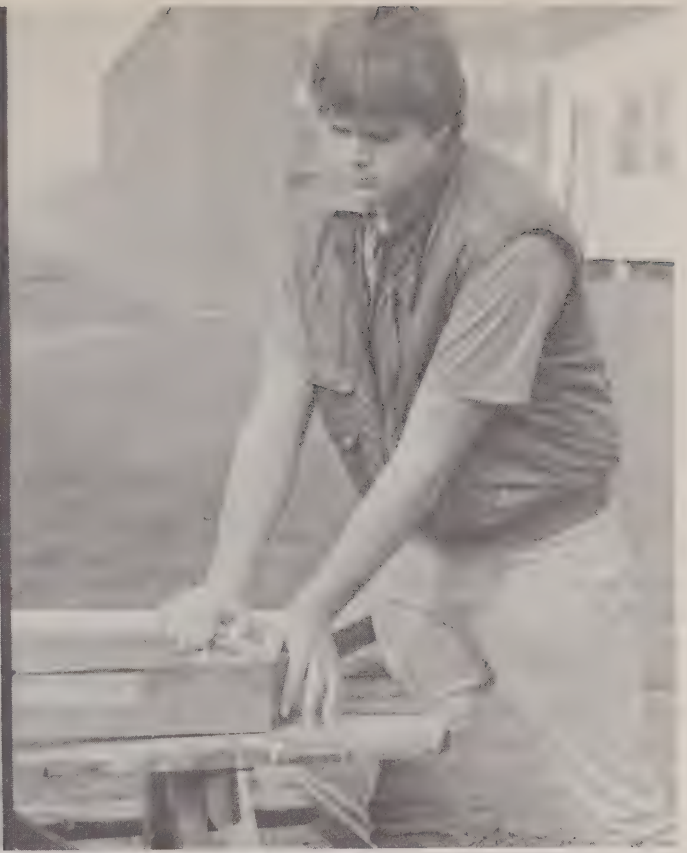
Matt Newton bolting together a frame.
