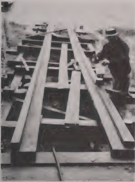
Charlie Burnham applies some grease to the launching rails.
