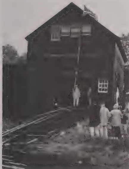
The flagpole/mast is raised into place prior to "Kim" emerging from the shop.
