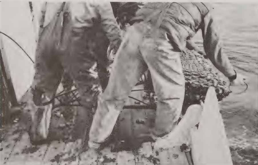
A gasoline engine (the winder) hauls the dredge aboard over the roller. Grabbing the large rings, the crew lift it onto the deck.
