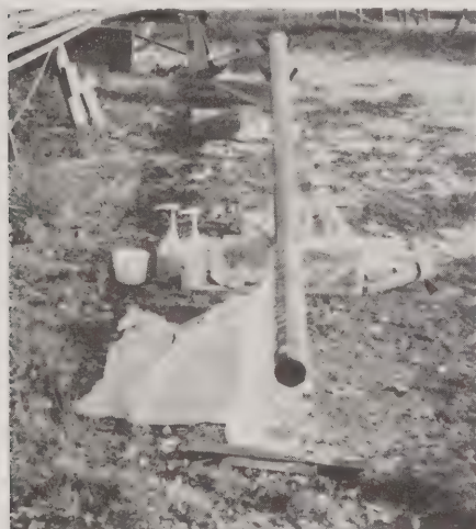
Fiberglass wrapping the top forty inches.
