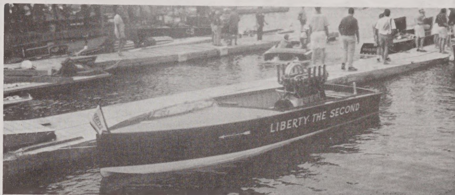
Liberty the Second , owned by the state of Pennsylvania, was raised in 1984 from the bottom of a Pennsylvania lake where she sank in 1922, and was claimed by the state from her salvors as being state property. She is powered by her original 8 cylinder Buick Liberty engine of 350hp.
