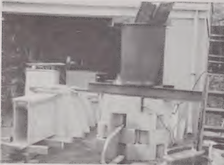
Melt underway, note fuel source, fuel feed tubes and vacuum cleaners for forced air. Three burners used to guarantee sufficient heat.
