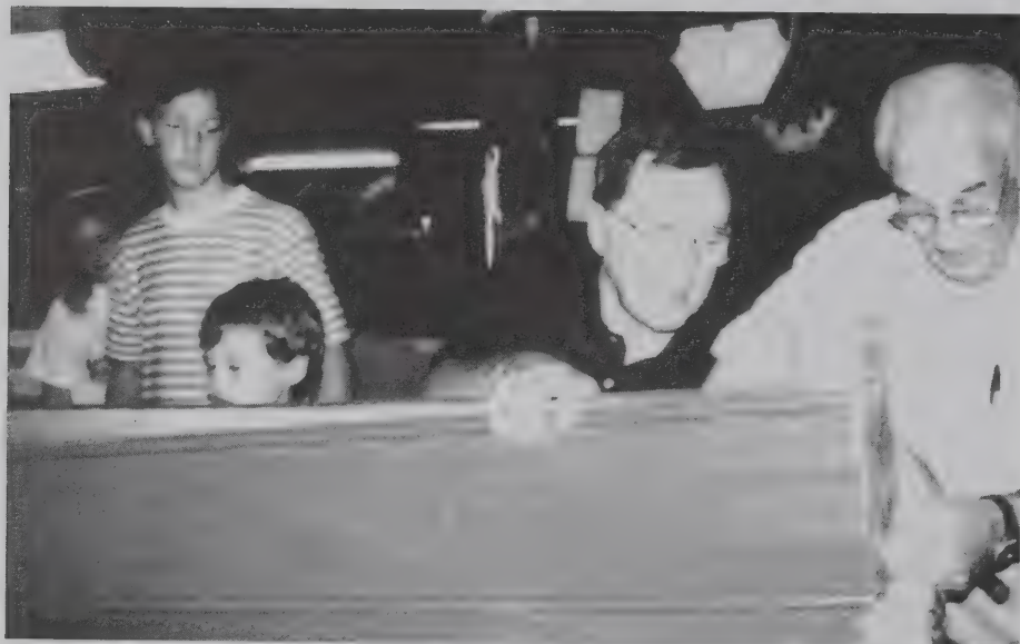
Peter and Charlie attaching the tin roofing to the wood stick (the bow stem) with self-tapping screws and a power drill. A heavy bead of silicone had been applied to the wood just prior to this operation. Sam, the designated test pilot, peers over the side with skepticism.
