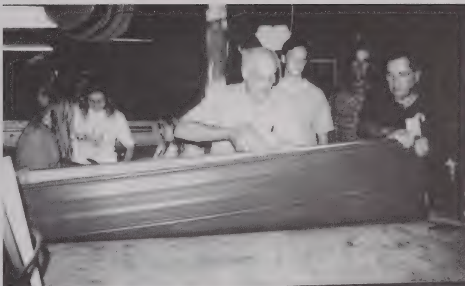
The final assembly is the insertion of the remaining piece of wood athwart-ship to provide a flair towards the bow.
