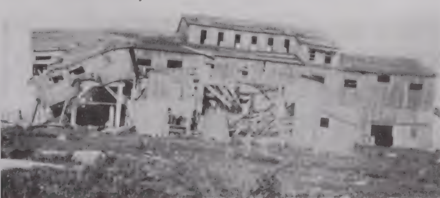
The old sawmill at Naubinway.
