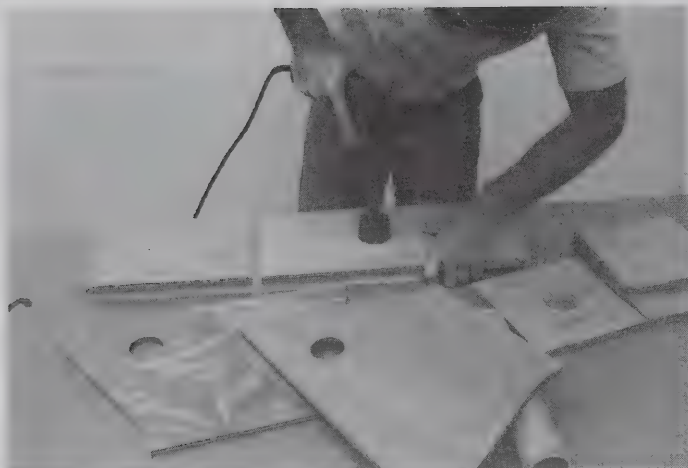
The plywood parts for the mount are laid out from patterns, sawn to shape, and holes pre-drilled as indicated.
