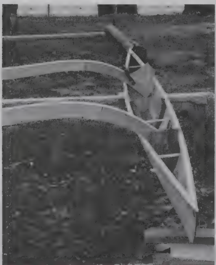
Setting up float hull.
