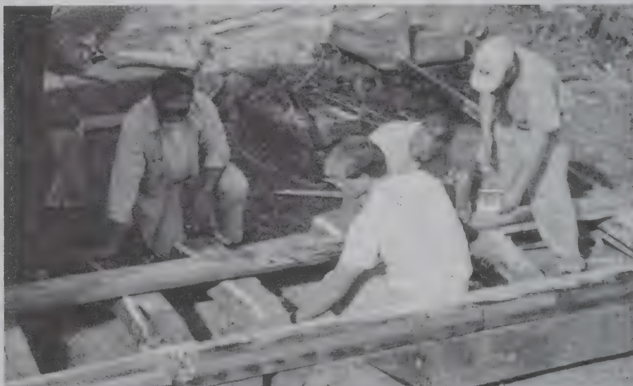
Lining up the keel rail under the stern, these volunteers are working to a string line set by the builder to assure parallel rails.
