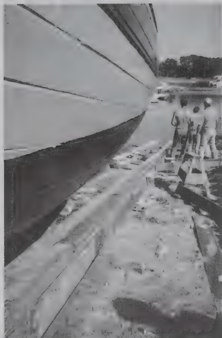
The Lewis H. Story is ready but the keel rail has yet to be completed up to the keel.
