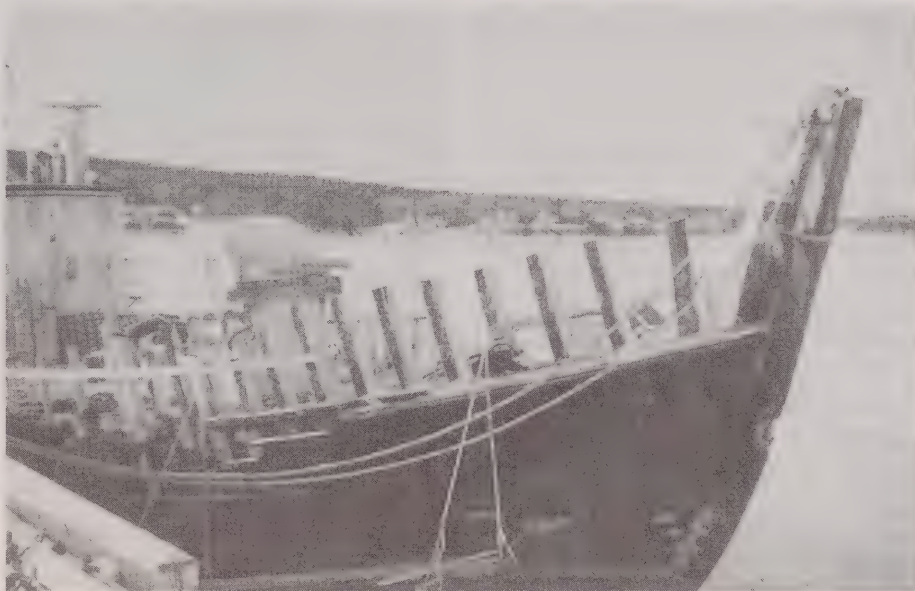
The refit begins with major timber repair and replacement.
