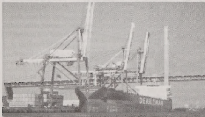
Typical river port scene, freighter terminal.
