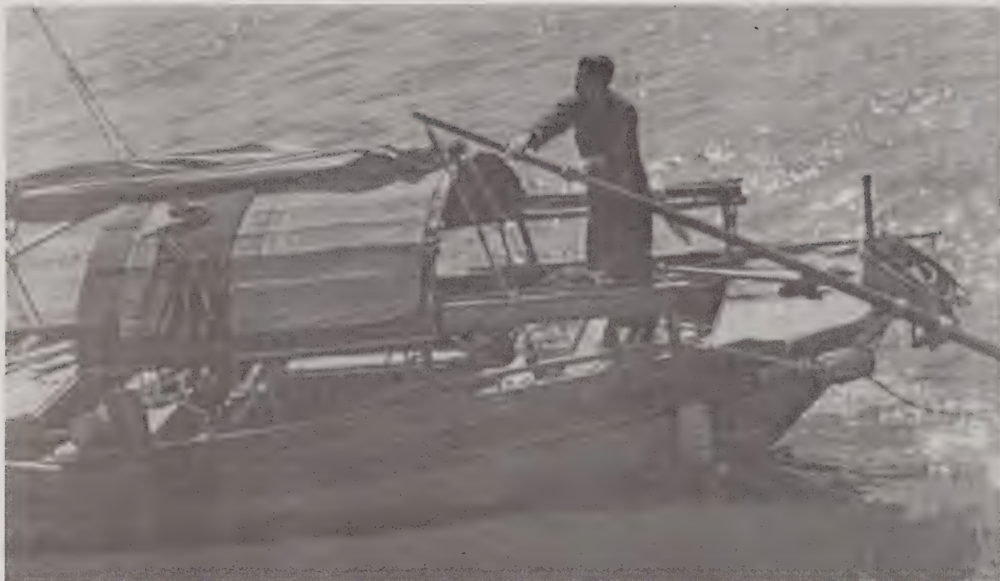
Photo found on an Internet auction site shows a very good view of a yuloh in use in the late 1940s or early 1950s.
