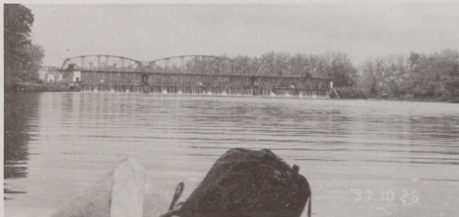
Approaching one of the dams on the Mohawk which regulate water level.
