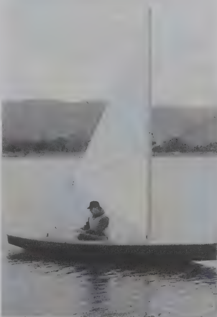
The June Bug mainsail is too small in light winds.
