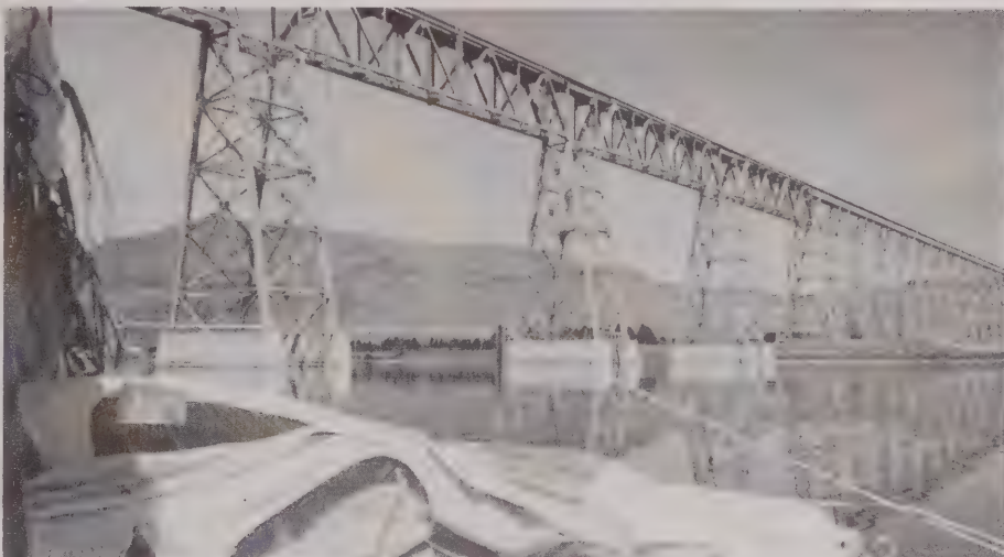
This railroad truss bridge offers 167' clearance. It was one of only three bridges spanning the Snake in 137 miles.
