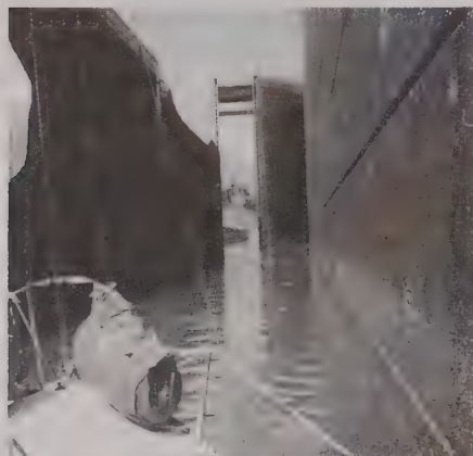
Lock swinging open at lower level.
