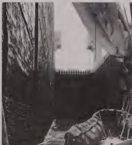
An intimidating prospect entering the guillotine lock.
