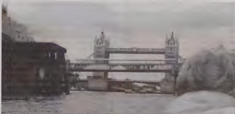
Tower Bridge coming up. To the left is the cruiser Belfast . The towers are joined high up with a fixed walkway, the roadway below it lifts for vessel passage.
