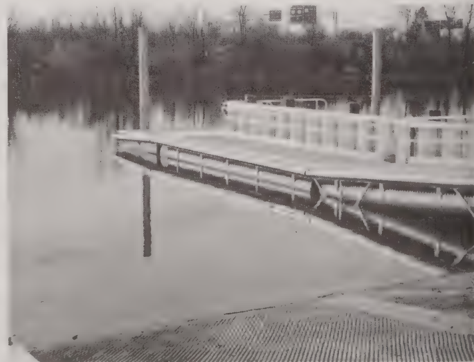
Floating pier at high tide (spring tide is about 6').
