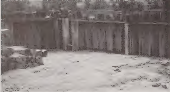
Build a steel wall around the area and pump it dry.
