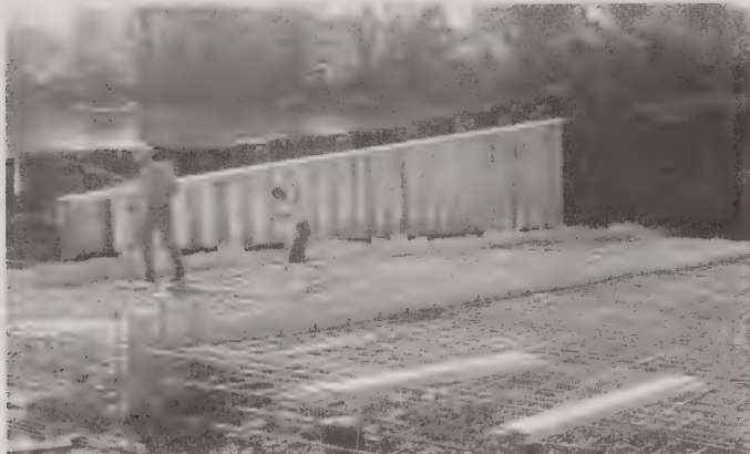
Lay gravel footings and reinforcing rods.
