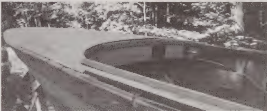
New deck in place awaiting new side rails.
