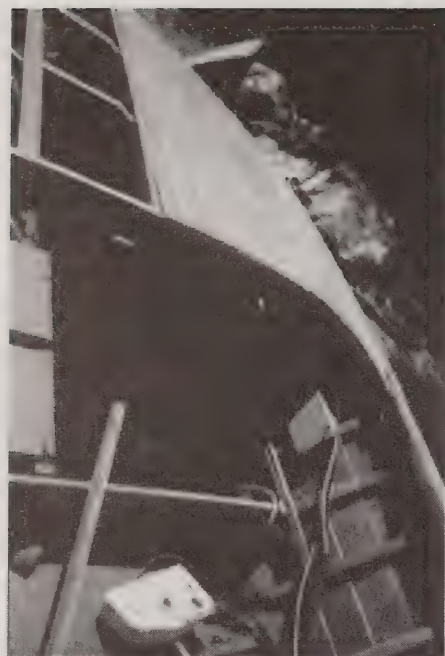
Half of the new deck going on.
