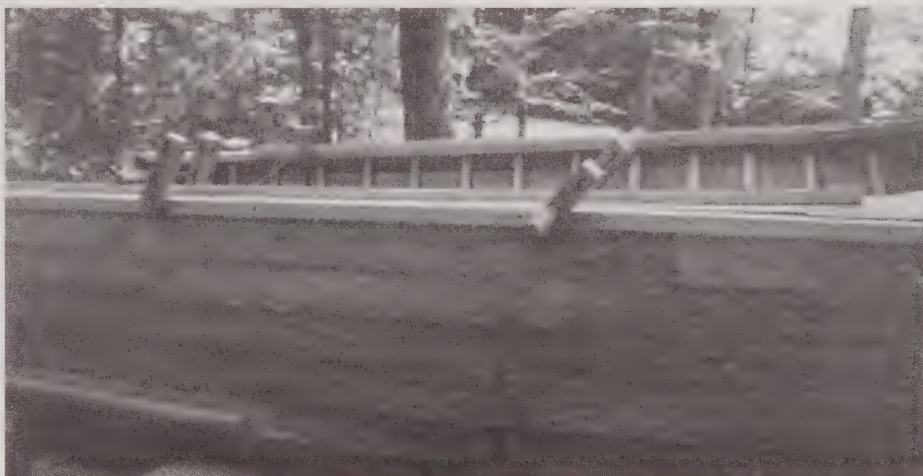
New side rails clamped into place.
