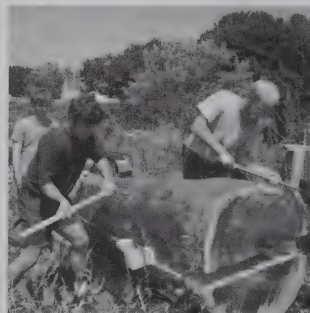
Apprentices hand-splitting, or 'hewing' the white pine logs used to create the frame mock-up of Red Jacket .
