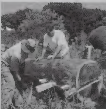
Apprentices hand-splitting, or 'hewing' the white pine logs used to create the frame mock-up of Red Jacket .
