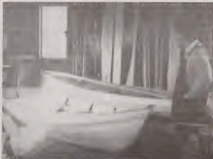
Albert (left) planes the bottom bevel to accept the garboard for one of the skiffs he built in his shop with son Bob (right) before his death in November 1951. Bob identified one of these skiffs in the collection of the Willowbrook Museum, Newfield, Maine. He donated the molds to Mystic Seaport Museum, and later, the plans to the Peabody Essex Museum in Salem (Robert H. Cloutman Collection).
