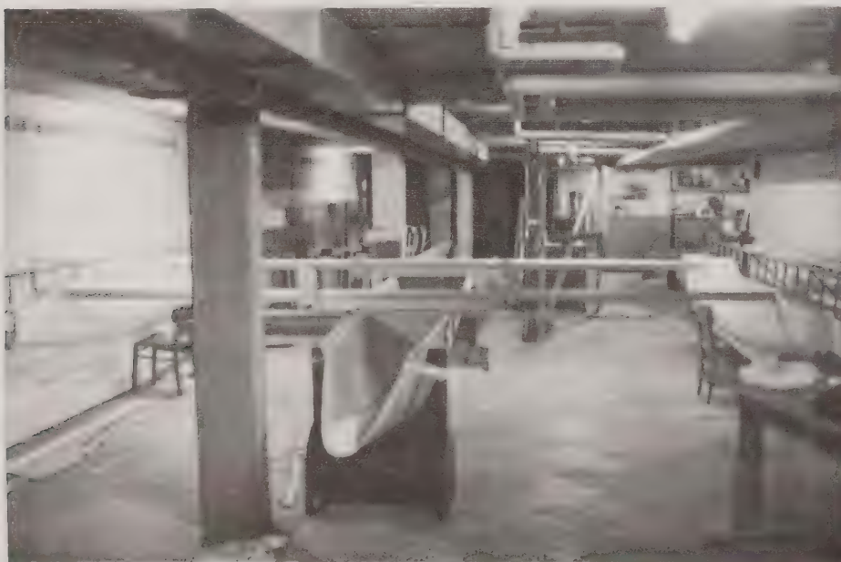
Mk. I under construction.
