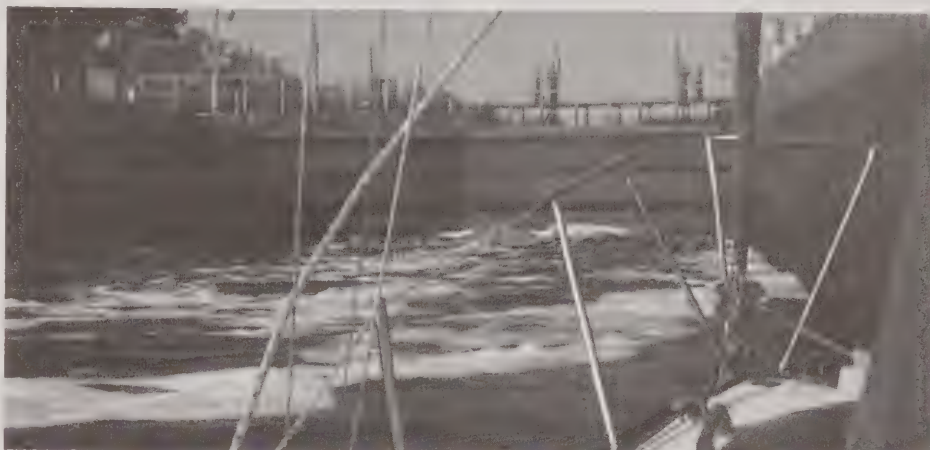
Deep Creek Lock being flooded.
