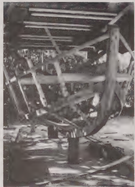
Frame up completed.
