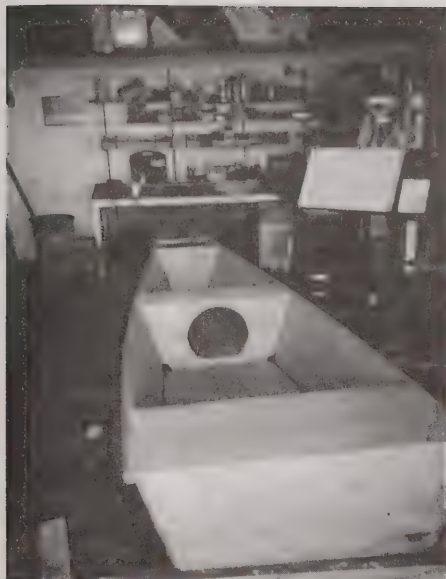
Half a schooner under construction.
