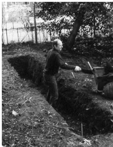
Digging the trench.
