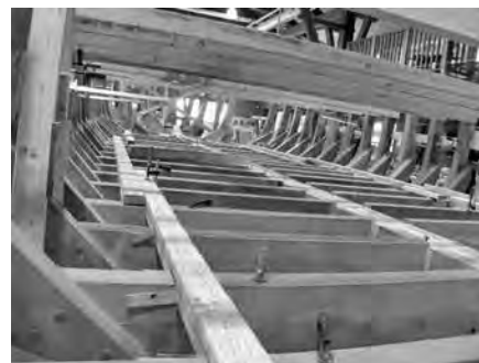
Inside the frames looking aft.
