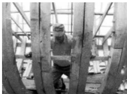
Jim Parmentier (left) checks the fair of the bilge clamp footprint with a batten. Working with shims and epoxy (center), Les Perry fairs the outside hull. Fairing often requires the removal of legacy screws before applying the plank. (Right) Jim employs one of the many forms of removing screws, a large pair of vise grips and some considerable brute force. Some were placed in green wood and are nearly impossible to extract.
