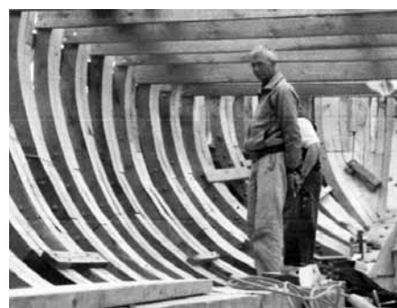
Dana and Gail survey the newly installed wedge clamps, heavy oak blocks securely bolted to the frame that are used to wedge the clamp planks into place.
