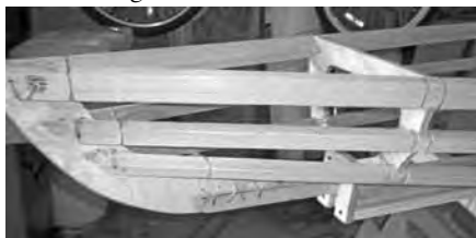
Deck beam lashed to first former.
