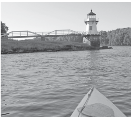
Doubling Point Light (Fiddler Reach).
