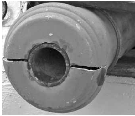
Steel pipe core and a fiberglass mask to look like a nine pounder for the movie, but aging ungracefully.
