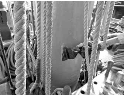
Yes, that is a weld, she carries steel lower masts.
