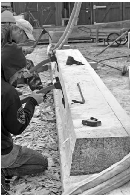
Shipwrights and apprentices use adzes to hand shape one of the nine logs selected for the historic restoration.
